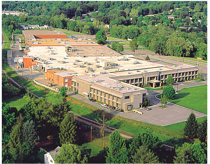
AERUS MANUFACTURING PLANT | BRISTOL, VA
